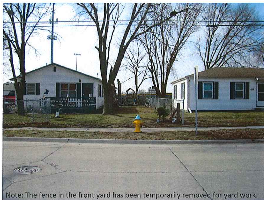
Below: Photo of the subject right-of-way facing South.
