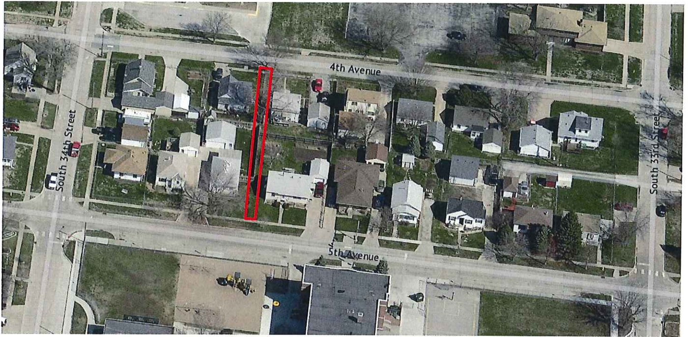
Aerial photo of the subject right-of-way (highlighted in red) facing north.
