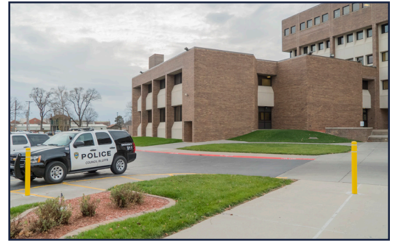
The current headquarters of the Council Bluffs Police Department
